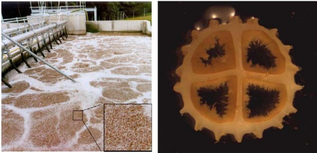
Figure 7 MBBR Carrier media in a MBBR tank
