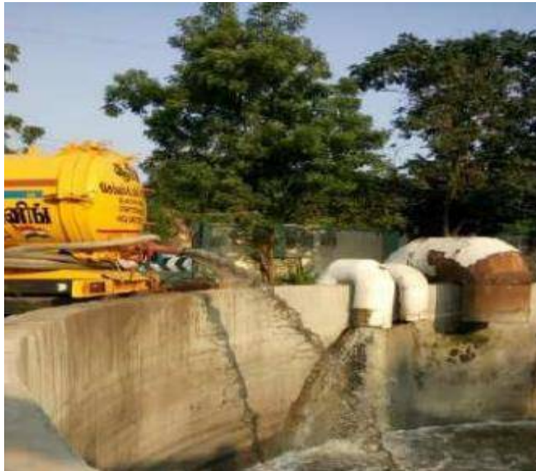
Figure 10Septage discharge using tankers
