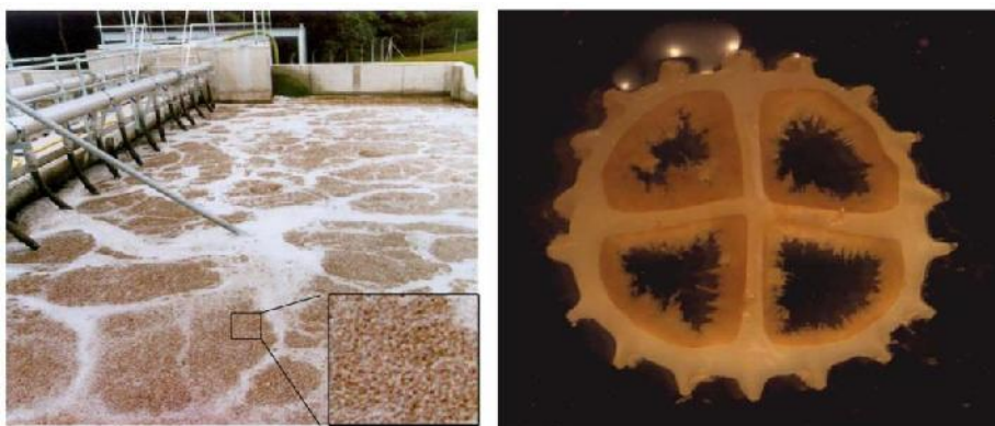
Figure 5.2 MBBR Carrier media in a MBBR tank
