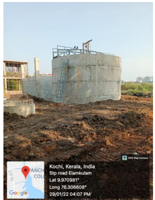
Fig- No.2.5 Construction of 5 MLD STP under AMRUT
