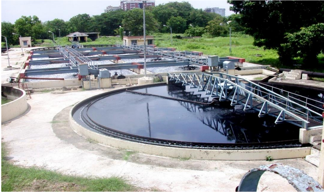
Fig.2.1 Existing Sewage Treatment Plant of 4.5 MLD capacity - Primary Settling Tank and Aerators
