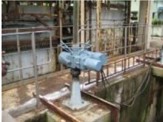
Figure 3.7 Electric motor driven gear actuator
