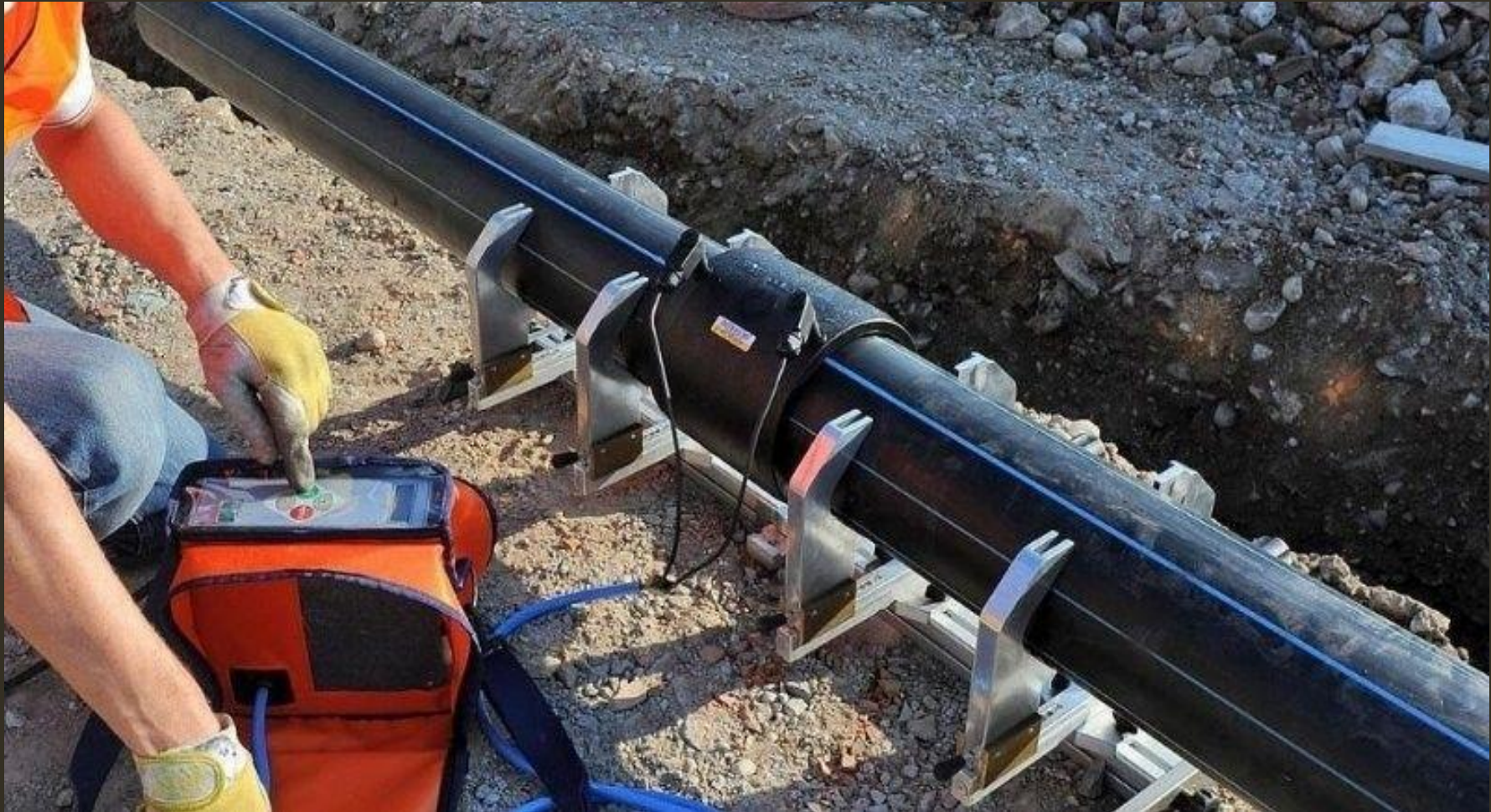
Electro fusion joint
