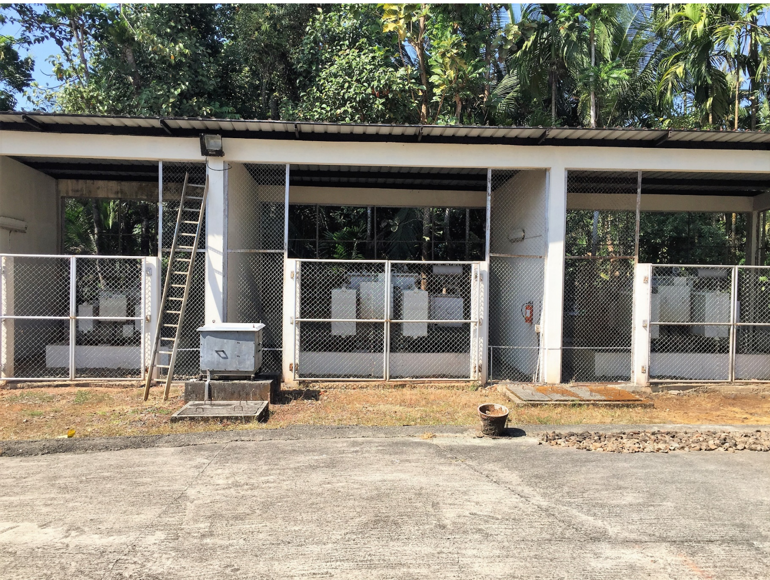
KVVA intake Pump house, Trivani
